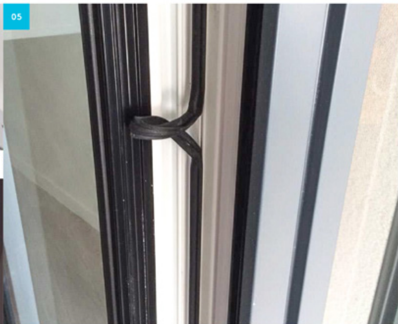
Change waterproofing seal
