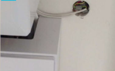
Install power cap on boiler
