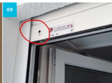
Install stop for rolling shutter
