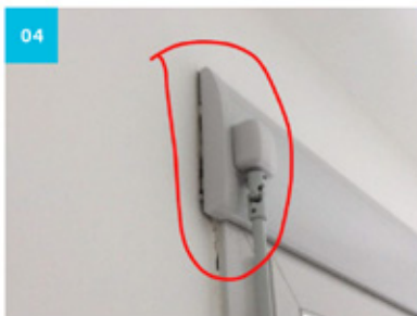
Install acrylic bead on the box
