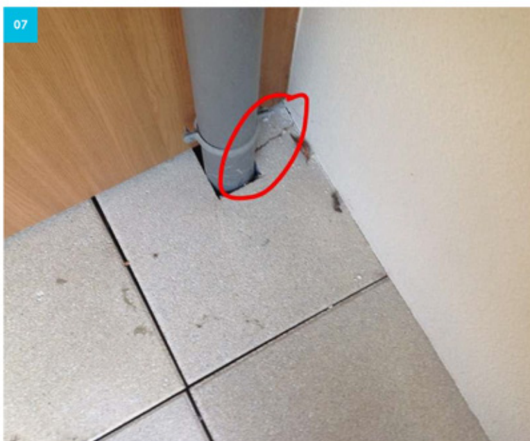
Redo slab around pipes
